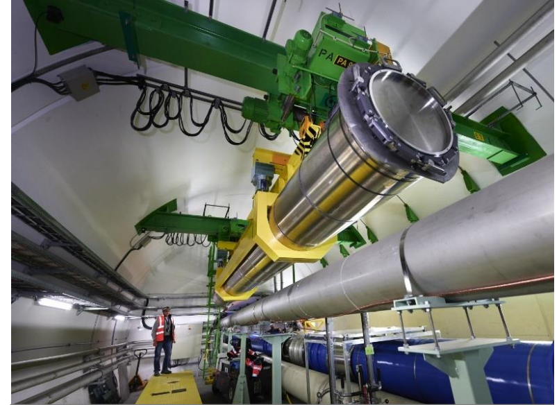
New dumps transport
