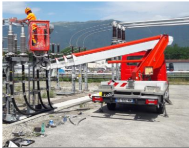
66kV Bus bars fixing
