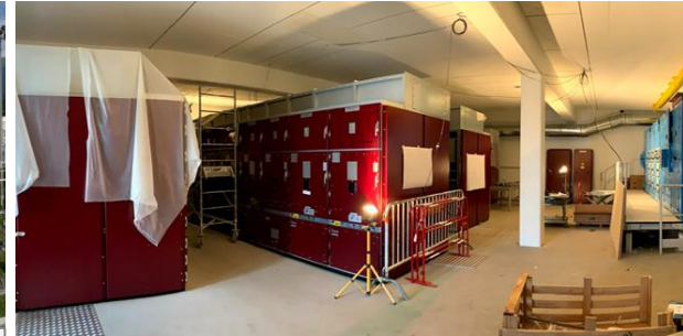
Primary 18kV substation -ME9/ consolidation & upgrade
