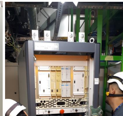
R2E: installation of new racks 600A
