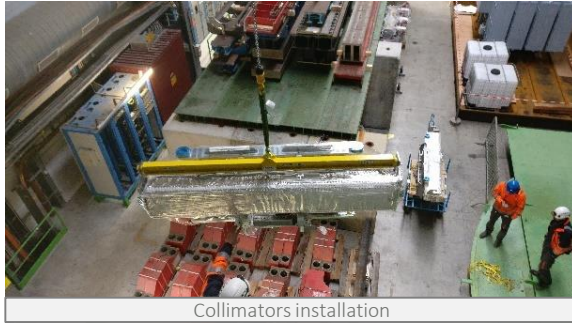
Collimators installation
