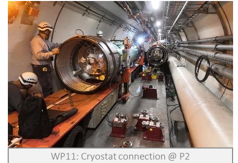
WP11: Cryostat connection @ P2
