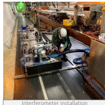
Interferometer installation
