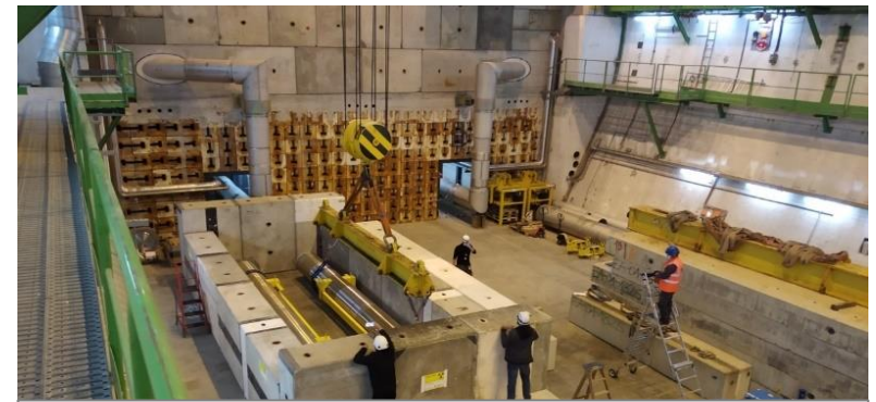
Ex-operational dumps store at UX65
