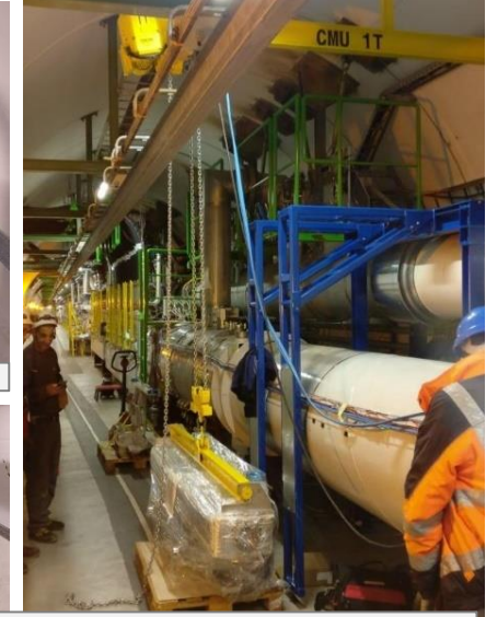
Collimators installation
