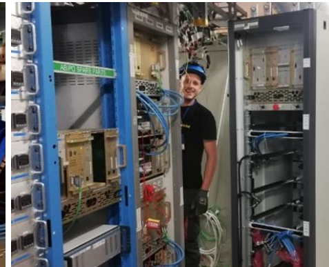
installation of new racks 600A
