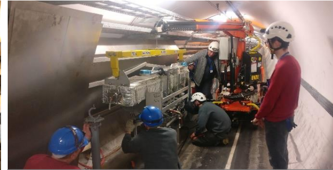
Collimators installation
