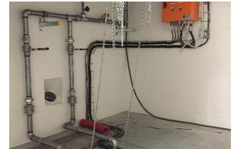
CV pump installation
