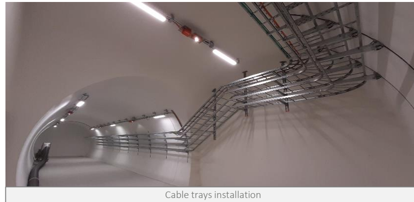
Cable trays installation
