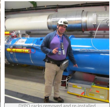
DYPQ racks removed and re-installed
