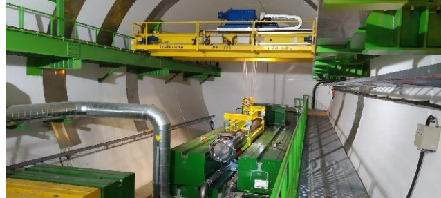
New dumps installation
