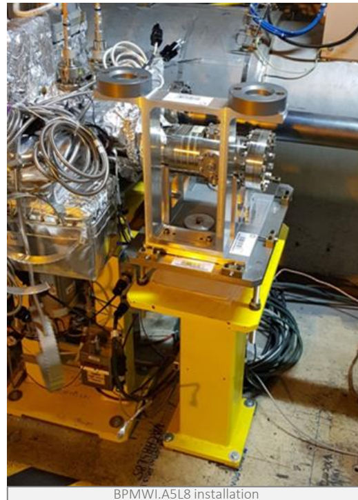
BPMWL A5L8 installation
