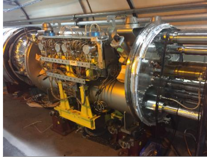
CC installation in P2
