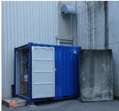
PAD-MAD PM25 upgrade works
