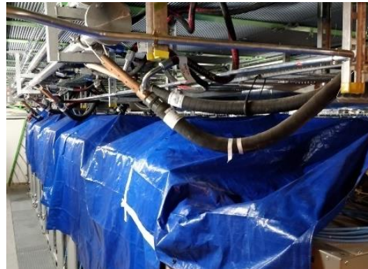
WCC hose replacement
