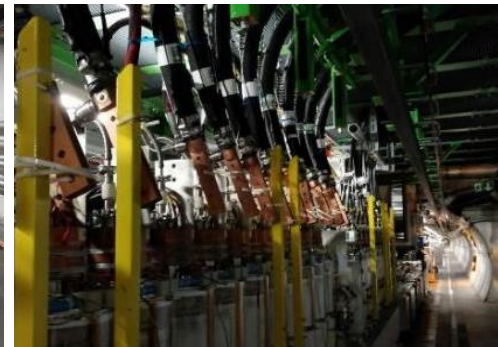
WCC hose replacement
