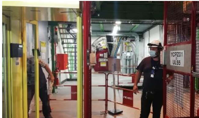
PAD-MAD UL55 renovation
