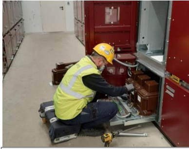
18 kV switchgear maintenance
