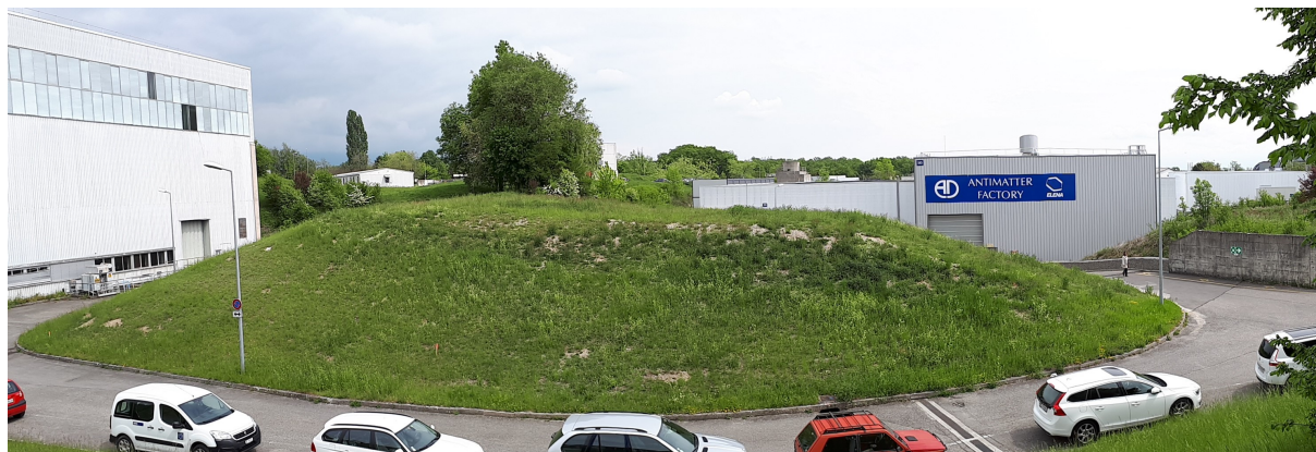
Figure 5.79: View of the proposed site looking north towards the existing earth mound.
