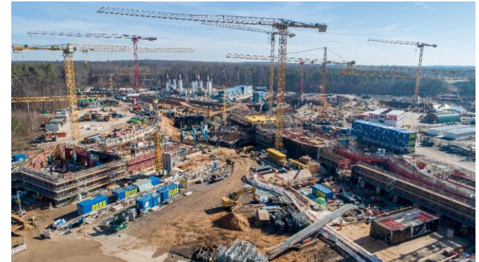
construction site FAIR, Feb. 2021
