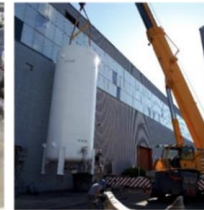
LN 2 storage tank - installation
