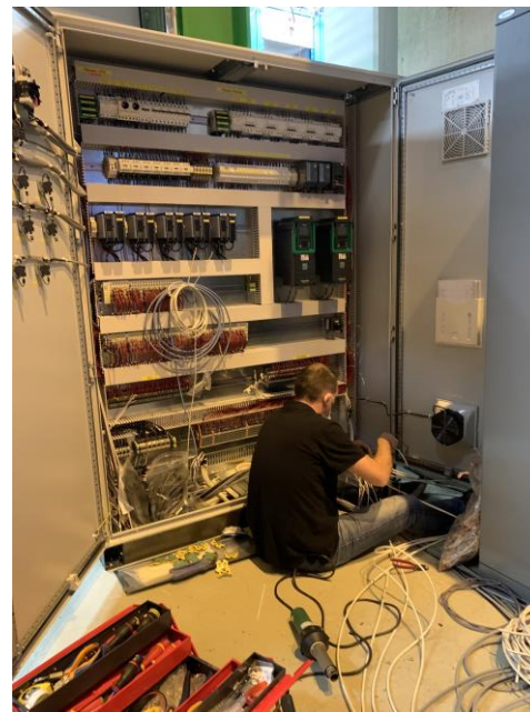
Cabinet cabling ongoing (EN-CV)
