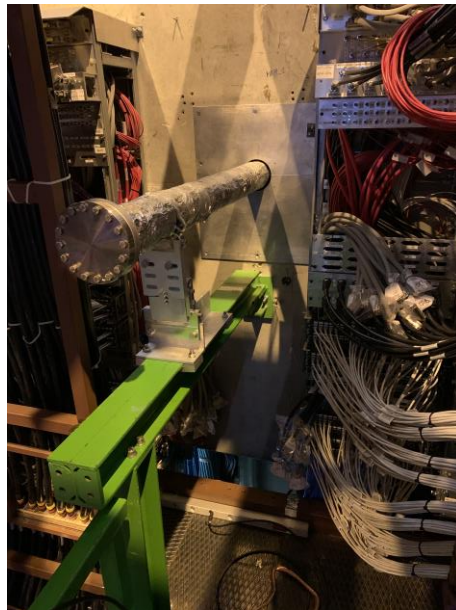
Installation 1/3 part RB24 beampipe
