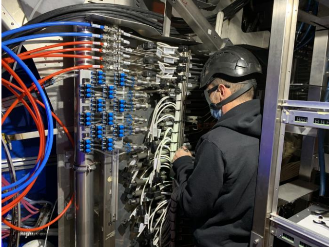
Installation pressure sensors, filters, manifold and valves
