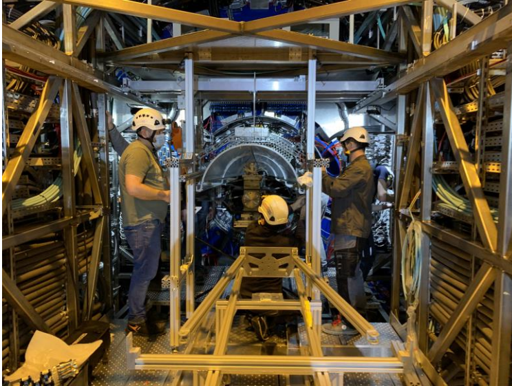
Handling test of the ITS chassis to simulate the installation of the Top and bottom ITS Half barrels inside the Cage
