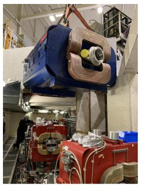
Work consists in opening magnets, replace shimming, check insulation, cooling, connectors, Perform measurement and certification
