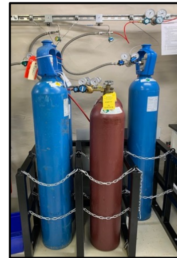
Gas cylinders (CO 2 , N 2 , O 2 ) used in biological sample maintenance are aged underground for a minimum of one month
