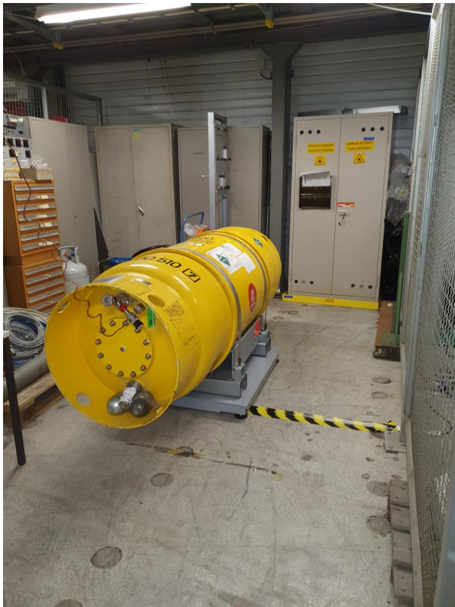
F2 chemicals bottle move in 888 R-024 next to RICH-1 Gas system
