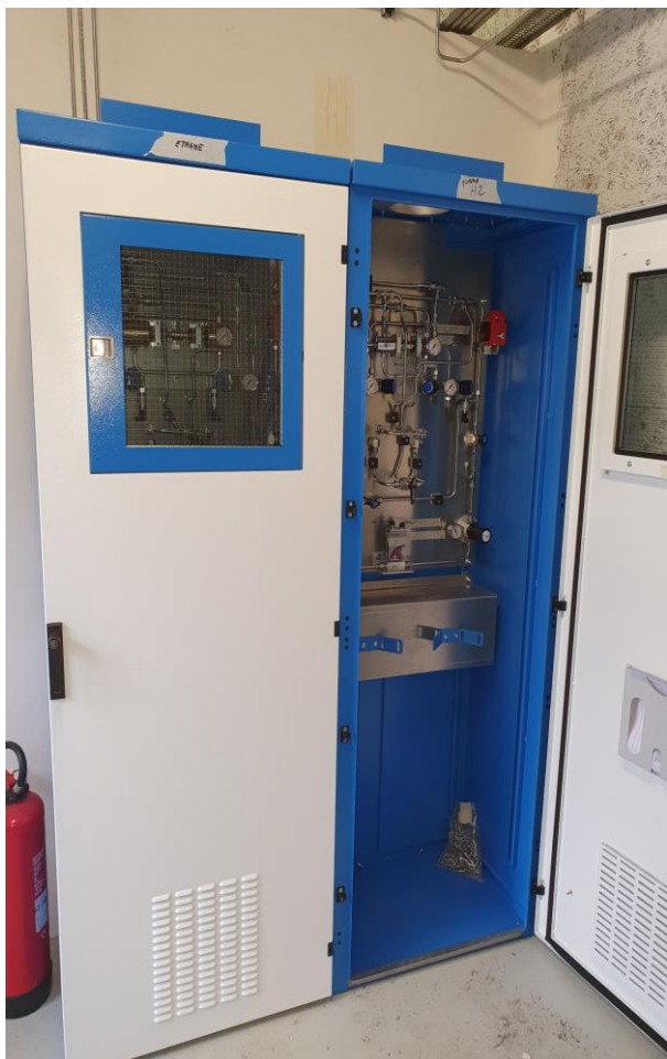
This Morning: Installation of the last rack for the methane bottle set
