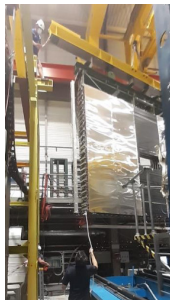
RW installation (June).
