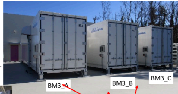
Capacitor Banks for BM3
