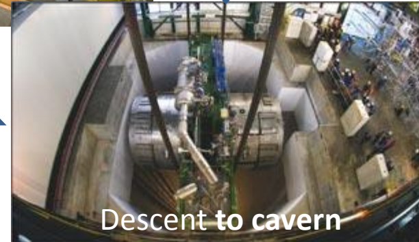
Cold mass rotated 90° and inserted
