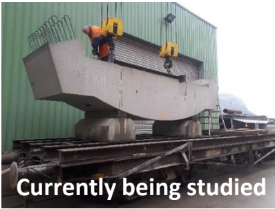
Pre-cast concrete invert (HL-LHC)
