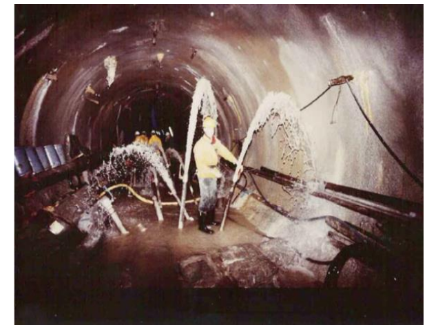
Water inflows during LEP construction
