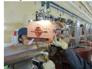
Installation of bellows chamber using crane
