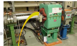
Cracked beam pipe (Al)
