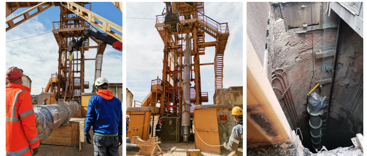
Test installation of the module
