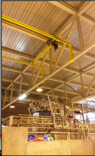
Installation of the WIZARD crane (courtesy: J.L. Grenard & team)
