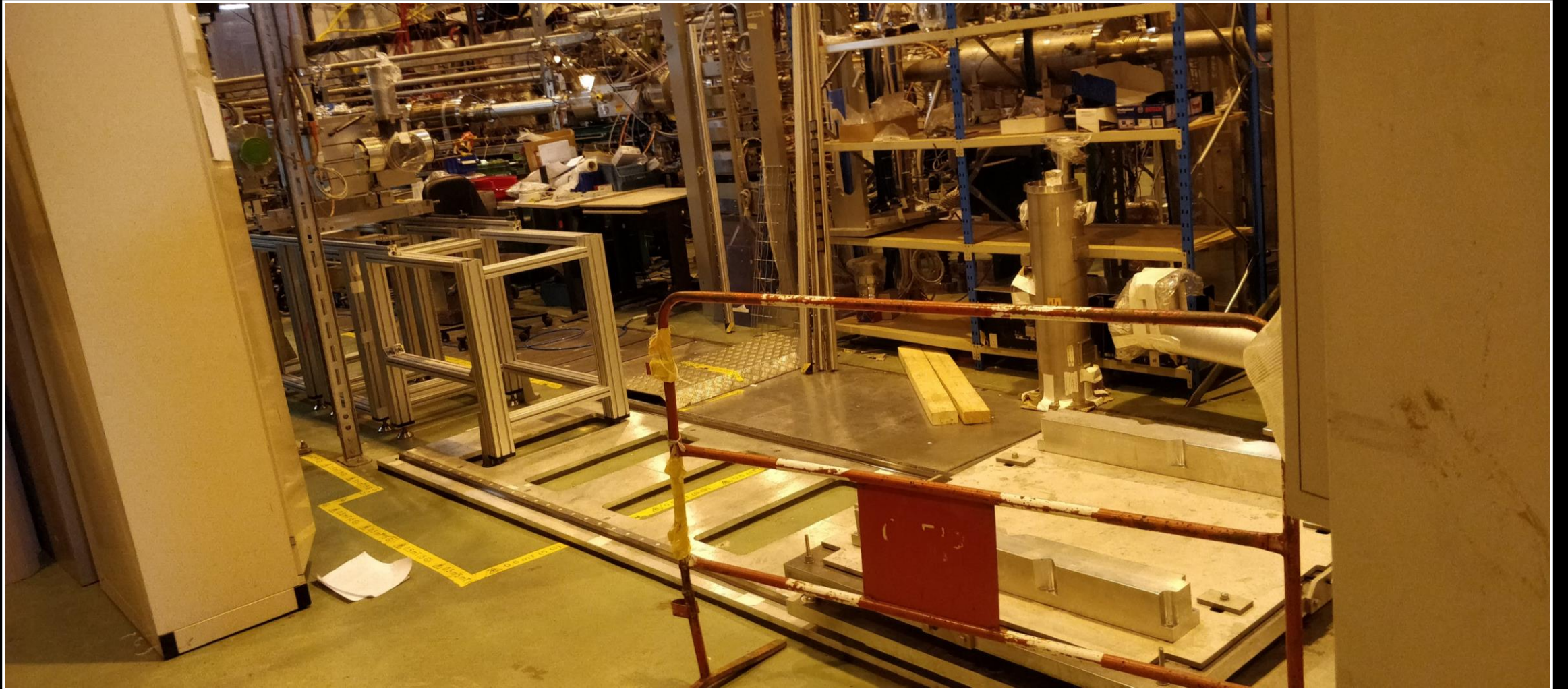
VITO: plates installed for easy moving of superconducting magnet. Due to arrive in March to hall
