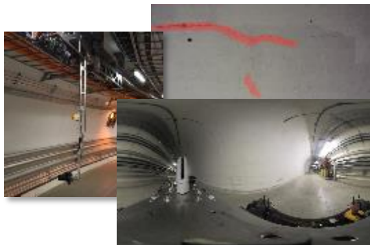
Tunnel structure monitoring
