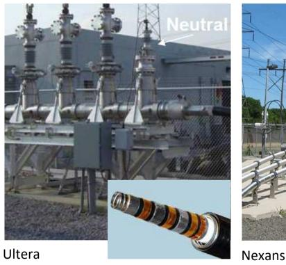
13.2 kV, 3 kA, 200 m Triaxial<sup>™</sup> Design BSCCO 2223 Energized 2006 High reliability
