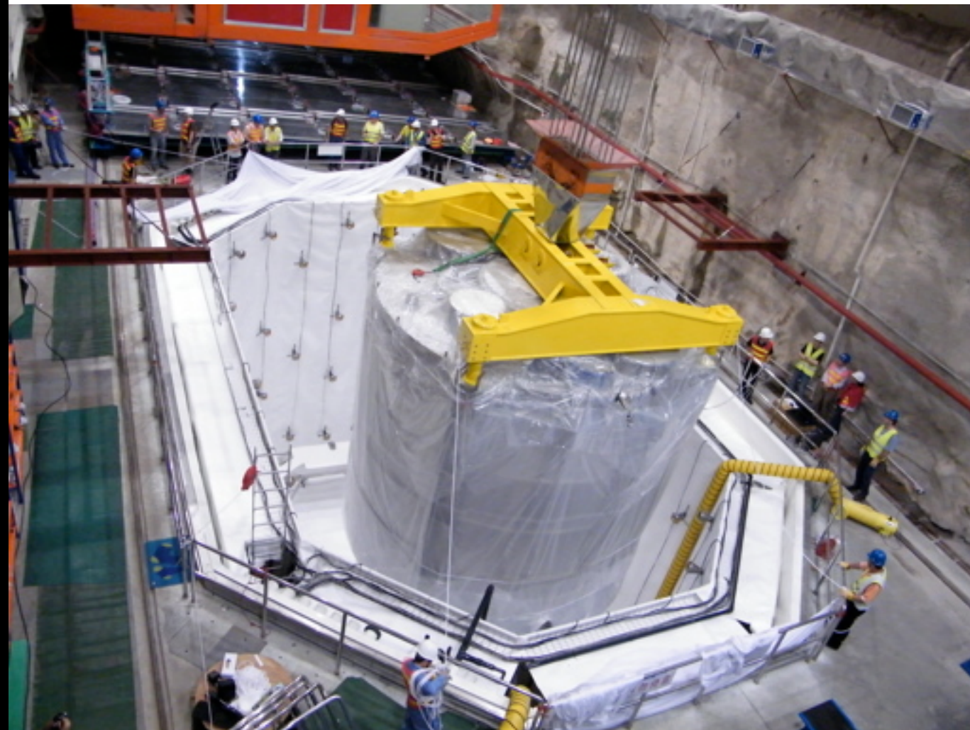
Installation of first AD at Daya Bay Site
